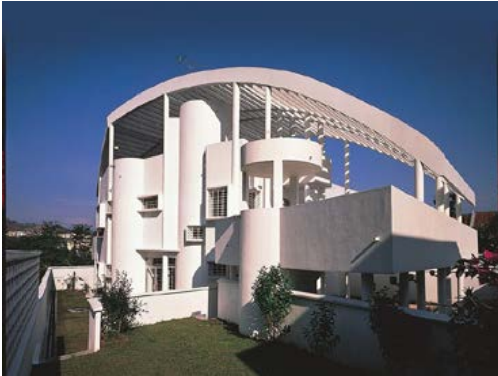
Roof-Roof House, designed by TR Hamzah & Yeang. The passive-mode, low-energy house was completed in 1985 in Kuala Lumpur
