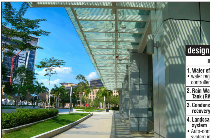
verandah with fritted-glass canopy
